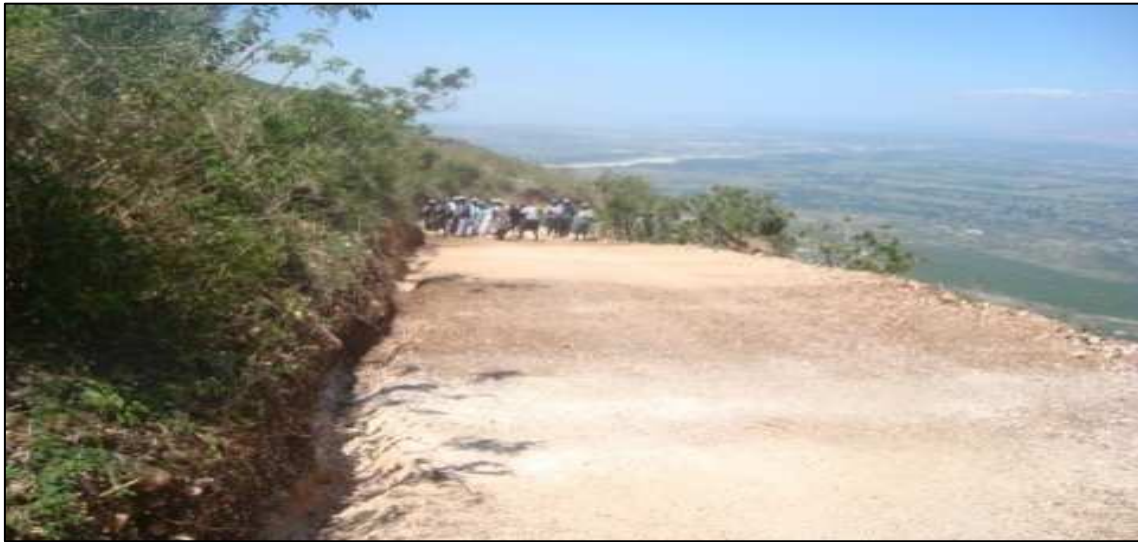
Figure 9-Road Rehabilitation works at Belle Fontaine and Zoranger in Croix des Bouquets.
