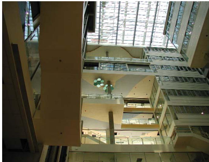
The Genzyme Corporation's recently completed office in Cambridge is a world-class example of green building construction, including advanced day lighting and thermal technologies. In addition to a photovoltaic installation funded by MTC, one of the most prominent features is a combined heliostat and reflective panel system designed to channel daylight deep into the 8-story building.
